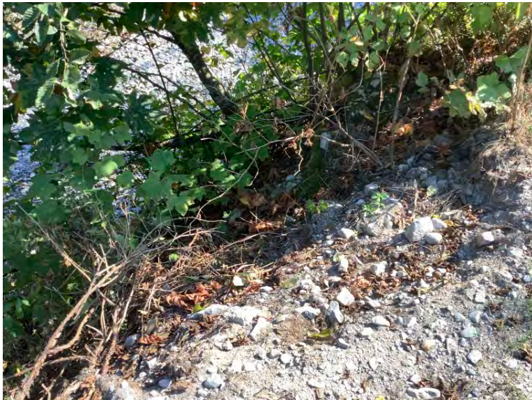
Left Bank Abutment when facing downstream
