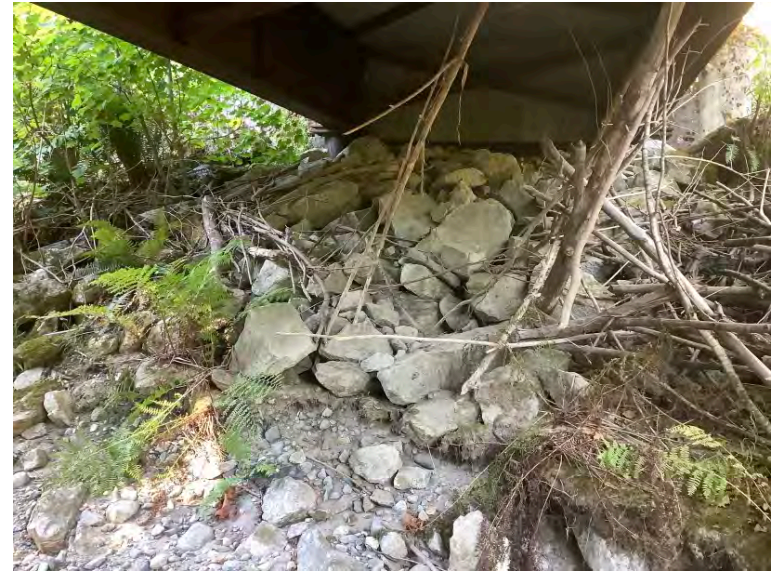
Left Bank Abutment when facing downstream
