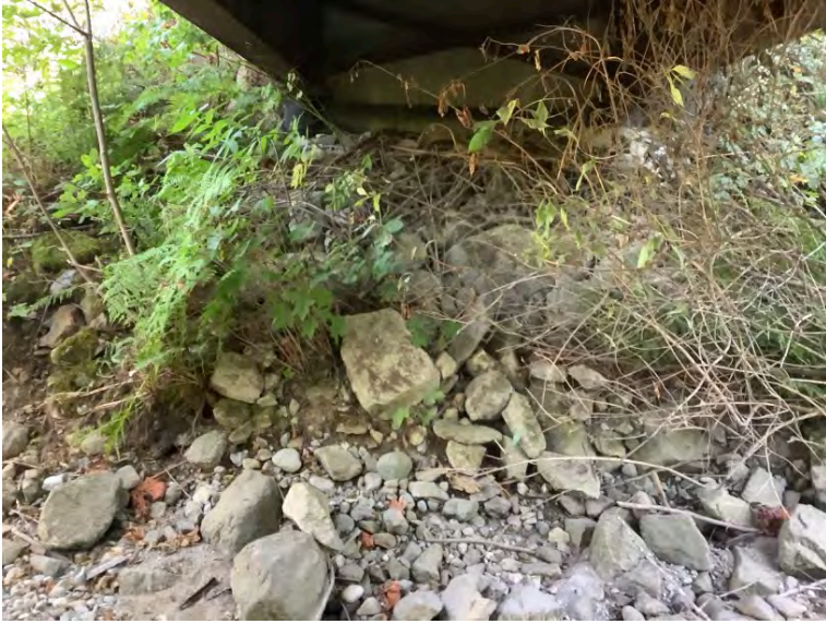
Right Bank Abutment when facing downstream
