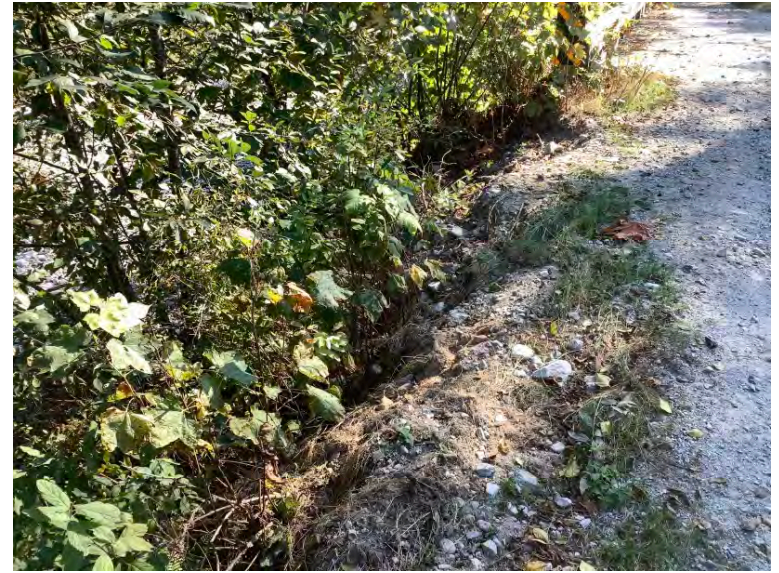
Left Bank Abutment when facing downstream
