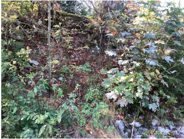
Left Bank Abutment when facing downstream
