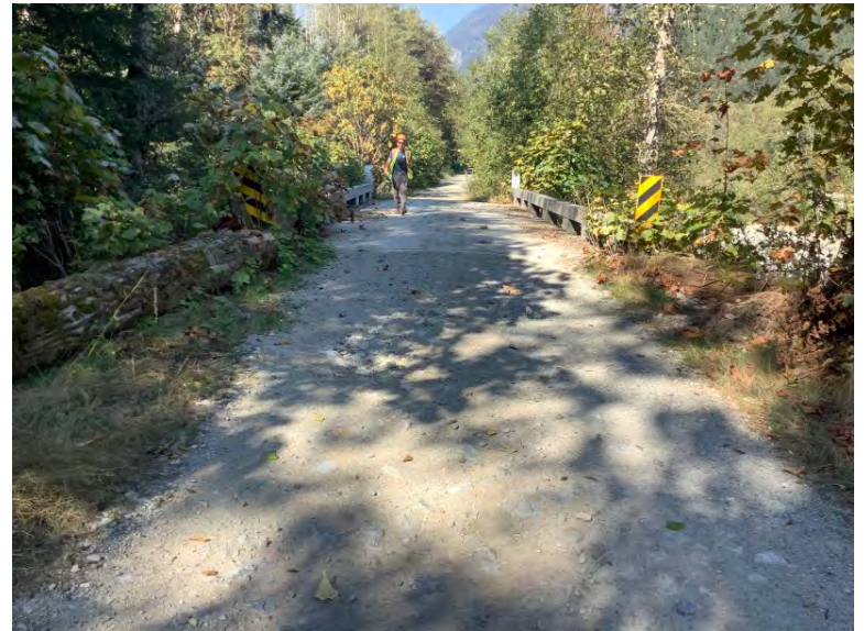
Right Bank Abutment when facing downstream
